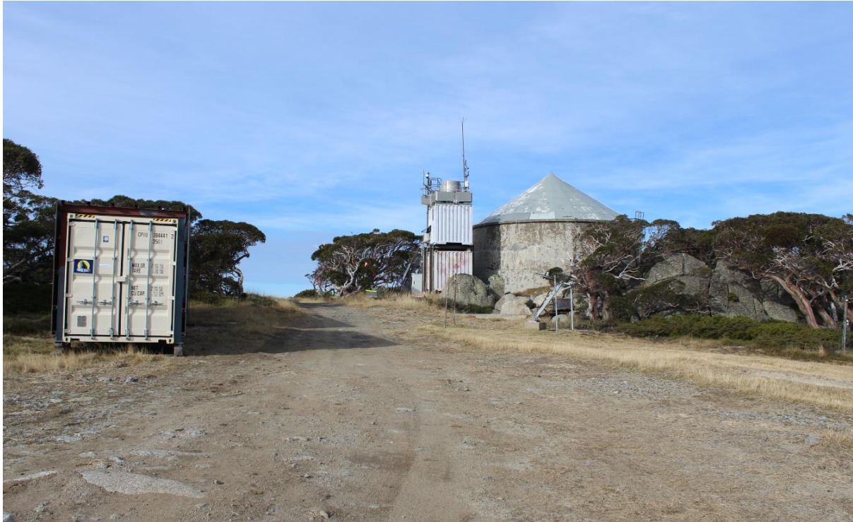
Figure 3: Existing portion of the access track from Blue Cow Ski building to be utilised by Optus for access
